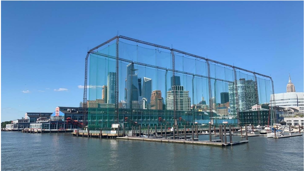
View of Subject Property from Hudson River looking northeasterly
