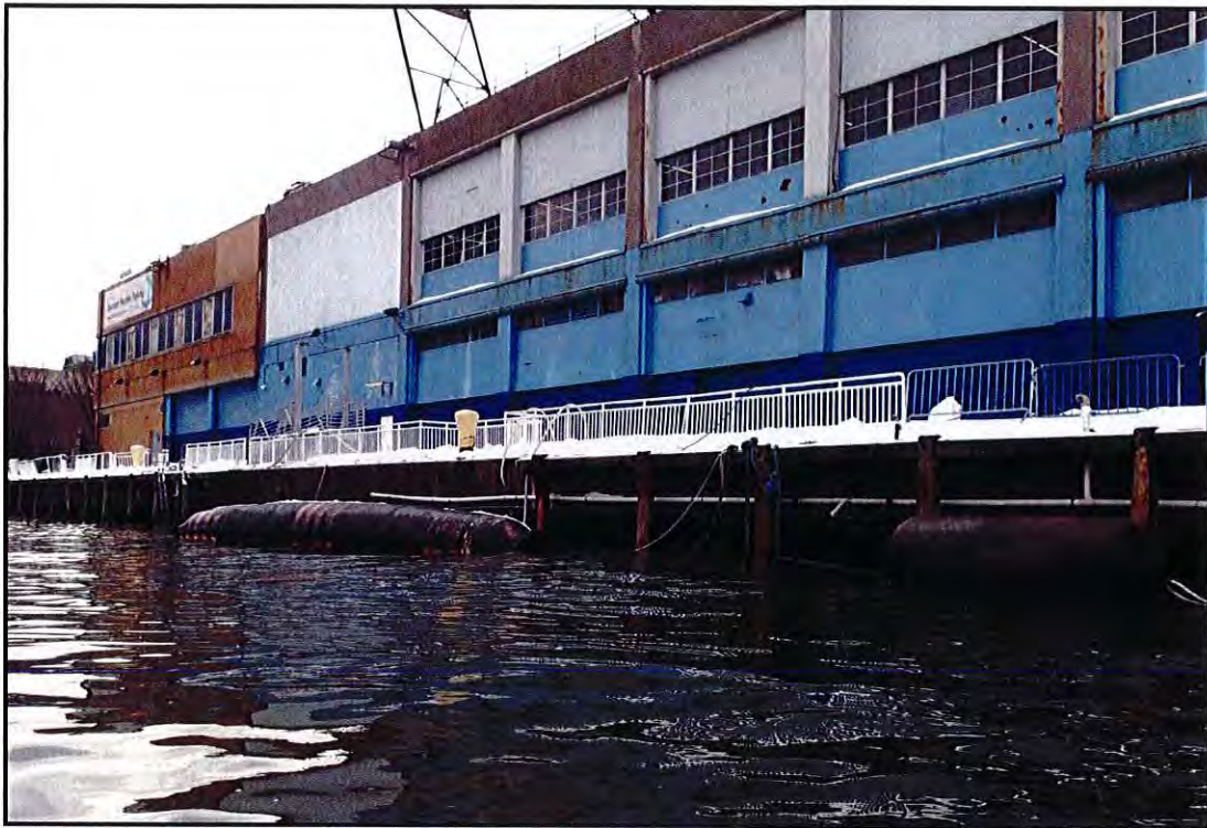
Photo B-7: View of north side of Pier 40 looking southeast. Note the timber fender system along the edge beam and additional floating fenders.
