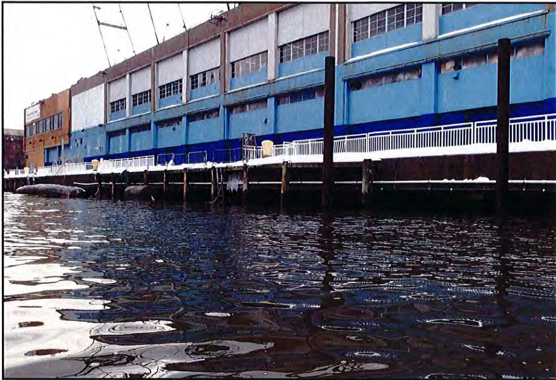
Photo B-39: Fender system along the north side of the Pier. Note the two steel fender piles located north of the timber fender system.
