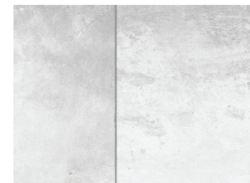
Concrete structural wall
