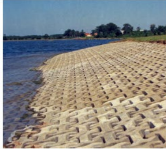
Revetments: Shoreline structures typically made of stone rubble or concrete blocks placed on a sloped surface to protect the underlying soil from erosion and reduce the force of wave action.
