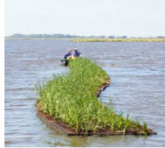
Floating Islands: Planted mats or structures that can reduce the impact of waves while providing ecological benefits, such as habitat restoration and improved water quality.
