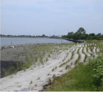
Living Shorelines: A bank stabilization technique that uses plants, sand/soil, and limited use of hard structure to provide shoreline protection and maintain valuable habitat.
