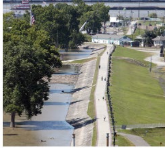
Levees: Embankments located at the shoreline that provide protection from flooding.
