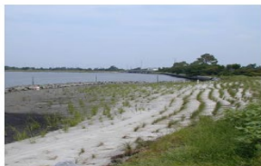
Living Shorelines: A bank stabilization technique that uses plants, sand/silt, and limited use of hard structure to provide shoreline protection and maintain valuable habitat.
