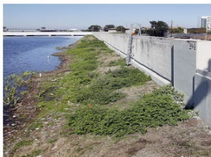
Floodwalls: Permanent or deployable walls used at the shoreline or upland to prevent flooding.
