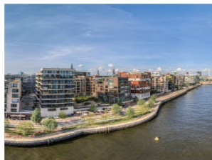
Elevation of Land and Streets: Elevation of existing or new development sites and streets above the expected storm level to protect from flooding
