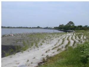
Living Shorelines: A bank stabilization technique that uses plants, sand/soil, and limited use of hard structure to provide shoreline protection and maintain valuable habitat.
