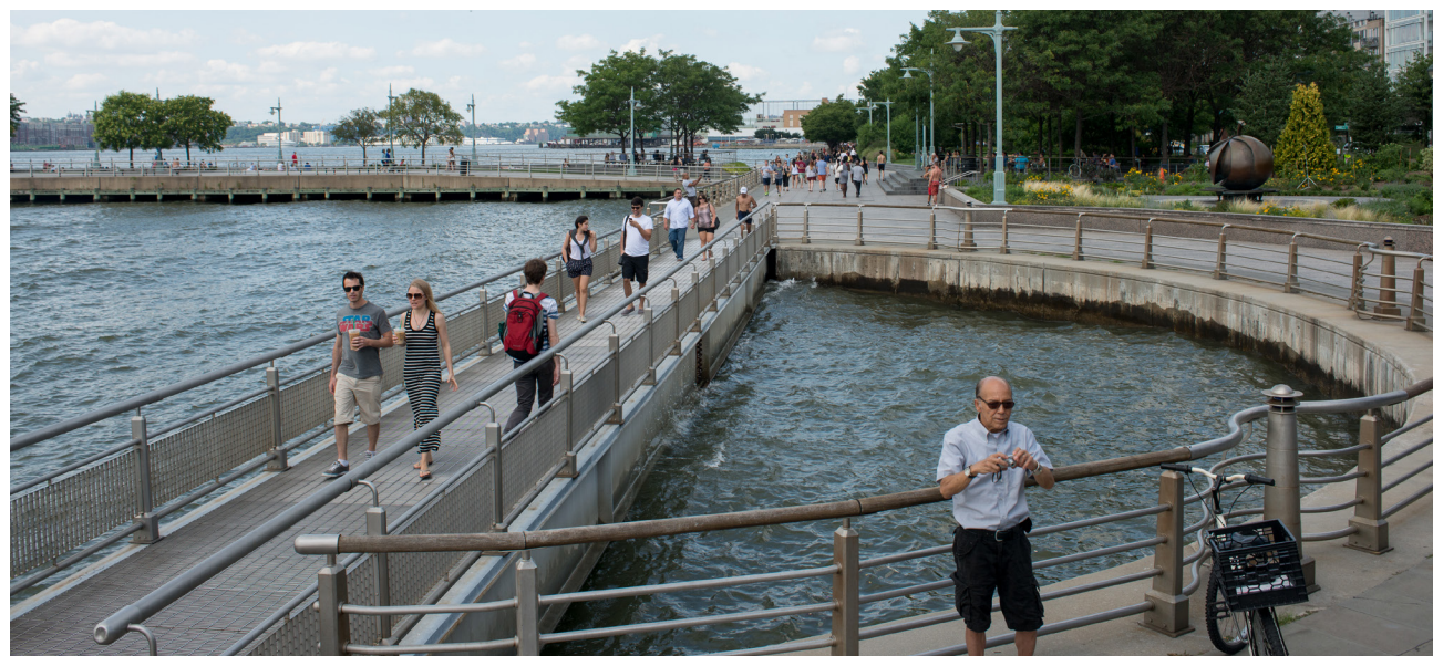
A bow notch located on the esplanade between Piers 45 and 46 in the West Village highlights an era of maritime history when, during the early twentieth century, port operators cut out notches from the existing seawall to accommodate larger and longer vessels.
