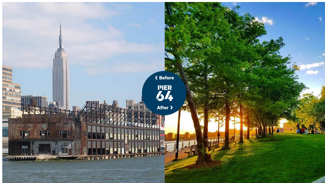
An area once filled with deteriorating steel beams is now lined with tall trees and shaded lawns. Pier 64 in Chelsea is part of the largest contiguous green area in the Park.
