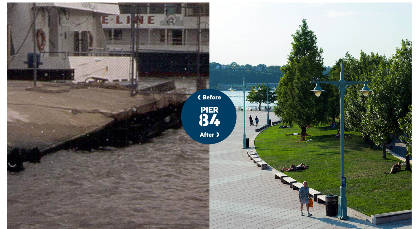
Rebuilt in 2006, Pier 84 stretches almost 1,000 feet into the River and measures nearly 100,000 square feet, making it one of the largest piers on the Manhattan waterfront.
