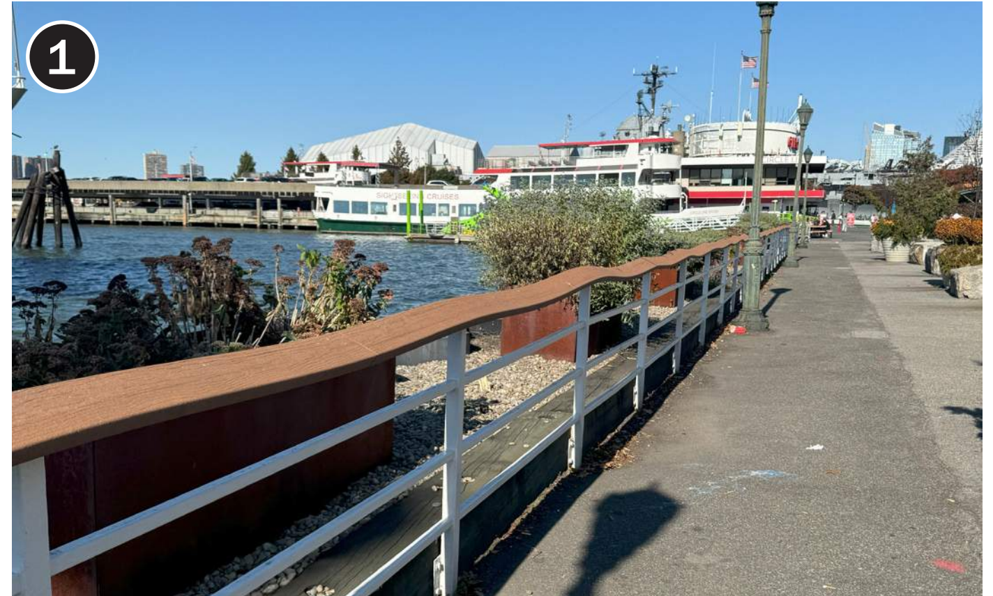
Temporary guardrail between Pier 81 & 83
